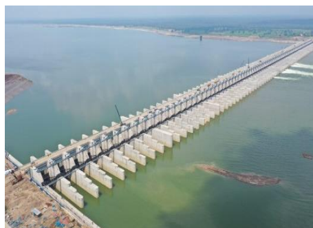
Figure 1: Lakshmi Barrage at Medigadda (KLIP)
